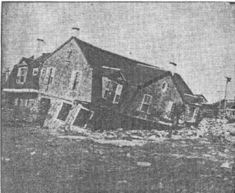
This large Summer home collapsed under the strain of high waters and wind. One entire section was undermined and the remainder is askew. This is another Westport Harbor scene.
