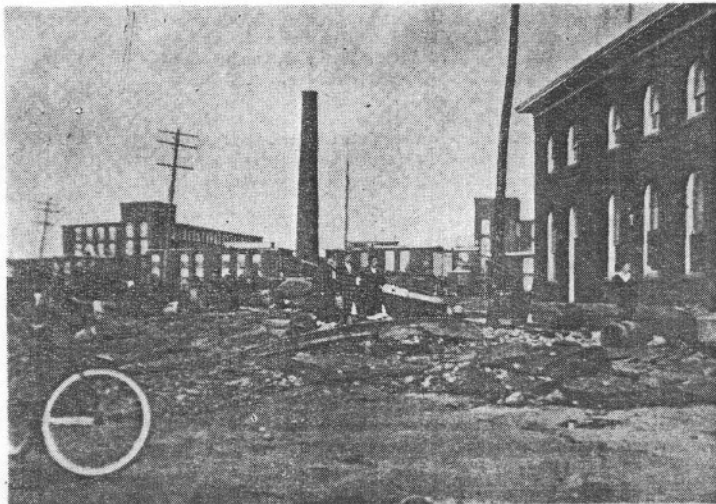
Residents view the wreckage on Cove Street after the water receded.
