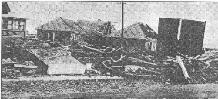
More damaged homes along the beach at Westport Harbor.
