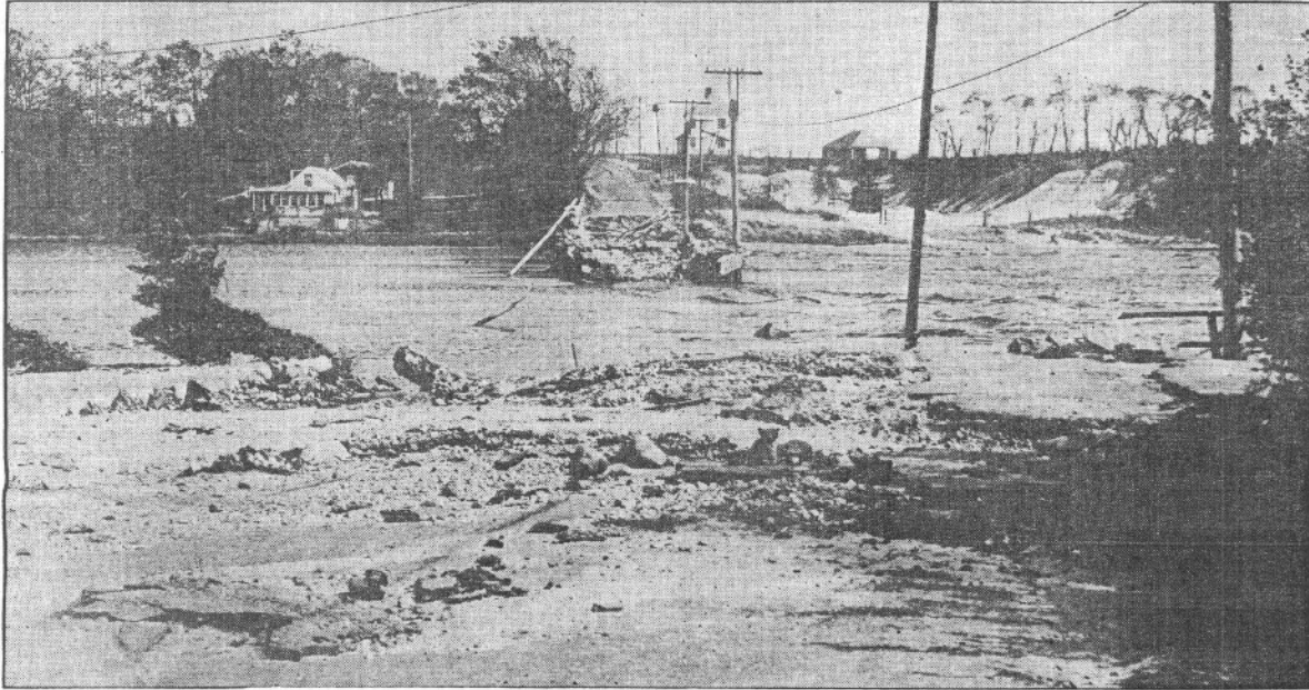
Hix Bridge was wiped out completely by the rushing waters. This picture, taken the day following the storm, shows nothing remaining except the bridge site.
